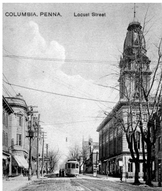
Looking east along Locust Street towards the intersection with Third Street. On the right is the Opera House, which in addition to being true to its name also housed the Borough office and small shops. In the left is Moses Bachenheimer's Clothing and Gent's Furnishing store in Eagle Hall. The trolley traveled around town on the same route its successor, Red Rose Transit, uses for its bus route.
