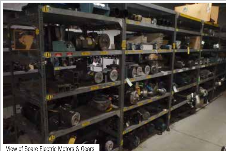
View of Spare Electric Motors & Gears
