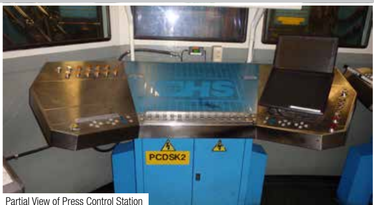
Partial View of Press Control Station
