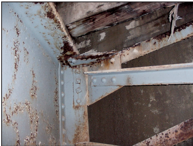
Figure 3—Chipping or flaking lead-based paint poses a health risk and may become an environmental contaminant. If field testing identifies lead in paint, a chip of paint should be sent to a certified lab for analysis.
